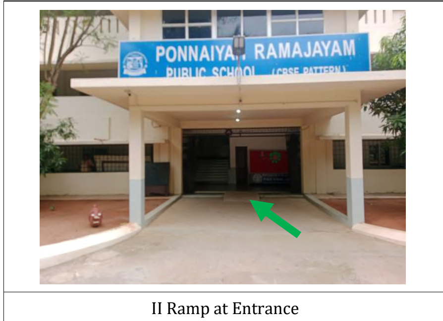
Photo. Ramps Facility
